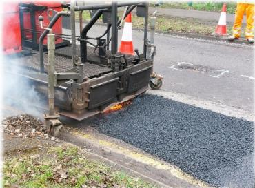
currently carried out using the Council's Rhino Patch resurfacing machine. As part of the review, the Select Committee conducted a site visit in March 2023 to see a reactive maintenance road surface repair using the Rhino Patch machine in Warren Road, Ickenham.
